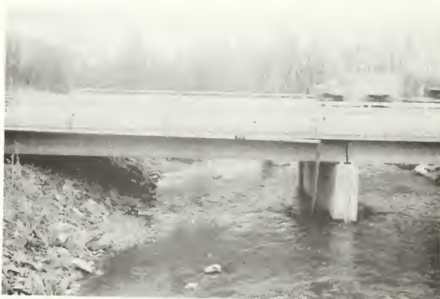
Boulder River Bridge Trail on 5/7/70
